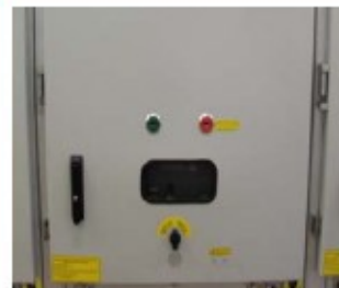
CB Compartment door with perimeter locks engaged
