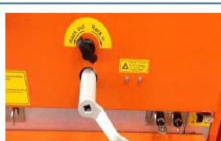
Manual racking handle inserted for operation
