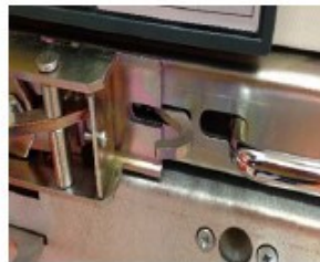
CB mounted mechanical hook
