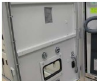
CB Compartment door open
