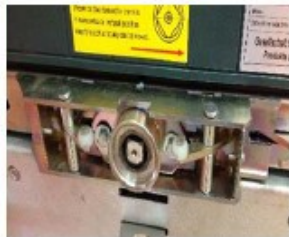
CB mounted roller actuator
