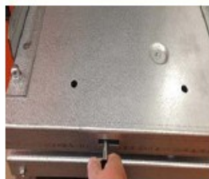
CB Trolley catch released
