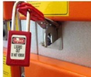
CB Lock operated and locked with personal padlock
