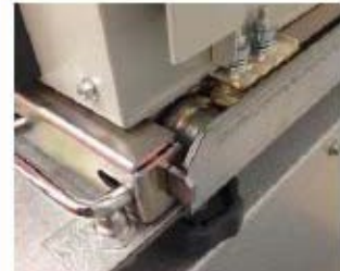
CB Truck RH locking pin in position on CB trolley
