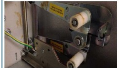
Shutter mechanism identifying padlock positions for both busbar & cable shutters
