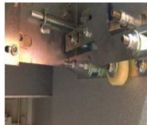
LV Plug Interlock mechanism in latched position
