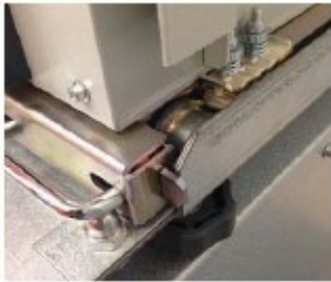
CB Truck RH locking pin in position on CB trolley
