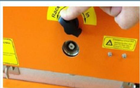
Manual racking access handle operated
