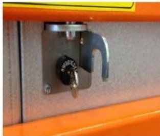
CB Lock operated and locked with key interlock
