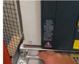
CB Truck LH locking pin retracted
