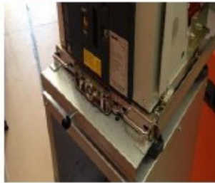
CB Truck locked on CB trolley
