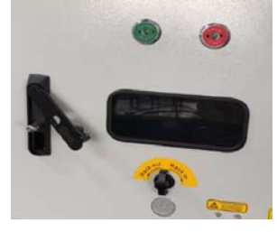
CB Compartment door rotated to open
