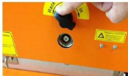
Manual racking access handle operated
