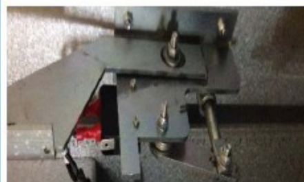
CB Lock mechanism (internal view with limit switch behind)
